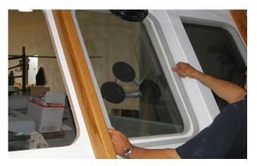
To install the inside molding, start by setting and fastening one corner at a time.
