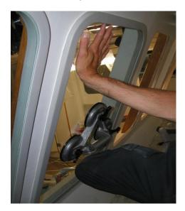
Place the window in the hole and have someone on the inside ready with small wood shims you have prepared earlier. The person on the inside will need to position the window in the center of the cutout and place shims at the bottom and possibly on the sides to hold the window at the most centered location.
